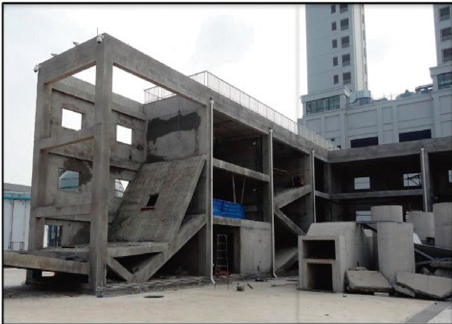
Escenario de Estructuras Colapsadas - Shanghai Fire Training Center, CN https://www.lionprotects.com/fire-training-structures/
